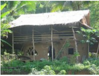
Almost finished our first mud house!!
