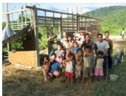
Building the kindergarten for Karen children at Nun's home
