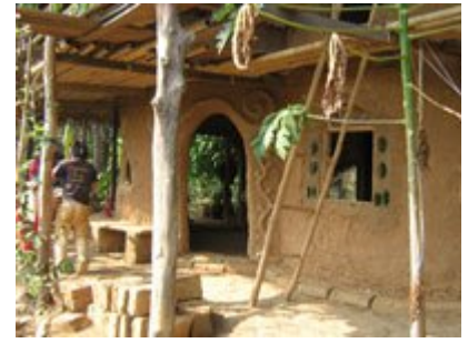
Ready to pain the earthen house.
