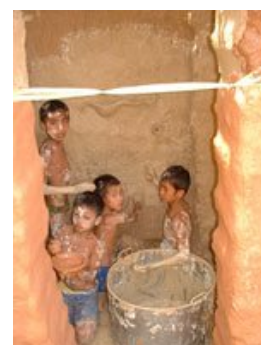
Painting the composting toilet with natural paints.
