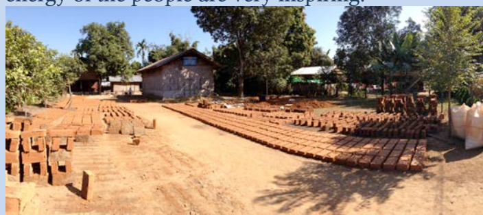
Mud bricks ready for the new kindergarten!
